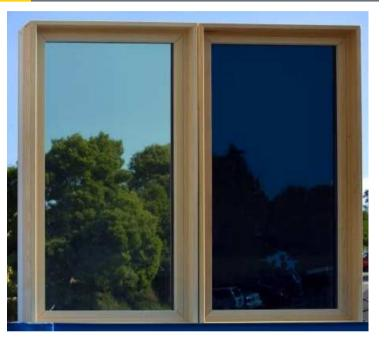
Prototype – Concept Window Highly Insulating and Dynamic U-factor 0.18 SHGC 0.04 – 0.34 Low cost unsealed center lite
